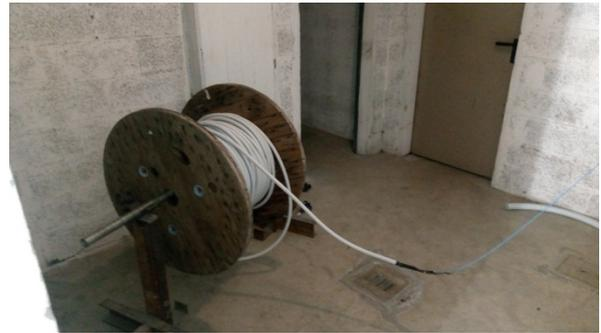
**Some pictures taken during the installation phase. The total length of the internal distribution grid was of 120 meters, passing through the cellars of the building.**
