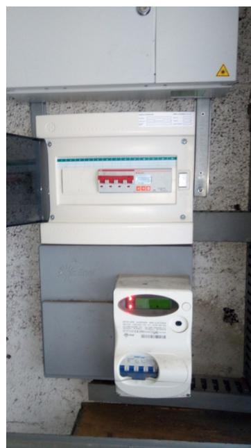
**Other pictures that detail the structure of the intervention. The first one is the main electric panel, equipped by the POD and 1 smart meter for the energy metering of 1 staircase.**
